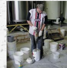
Mixing AQUAFIN ASODUR®-SG2 in supplied container.
