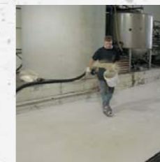
Application step 3, sanding of surface for bonding of subsequent epoxy top-coating.
