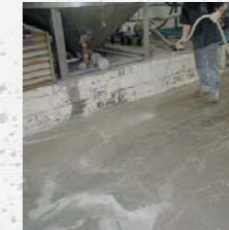
Cleaning / rinsing surface from debris.
