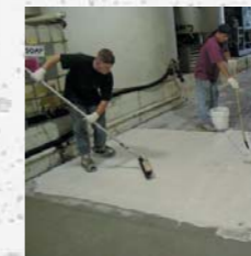
Application step 2, scrubbing material into the substrate pores with a brush.
