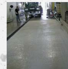
Finished surface, ready to receive top-coating.
