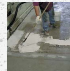
Application step 1, spreading material evenly over surface with squeegee or roller.
